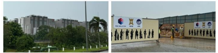
Figure 4: (L) GDS – early hyperscale DC in Johor at Nusajaya Tech Park; (R) IJM-Woh Hup DC construction at Nusa Cemerlang
