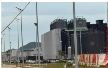
Figure 3: Construction works at YTL Green Data Center
